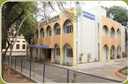
Dept. of Electrical Engineering
